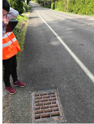
Photo 10 (looking N): Type 2 CB (#4). Inlet from 12" concrete pipe.
