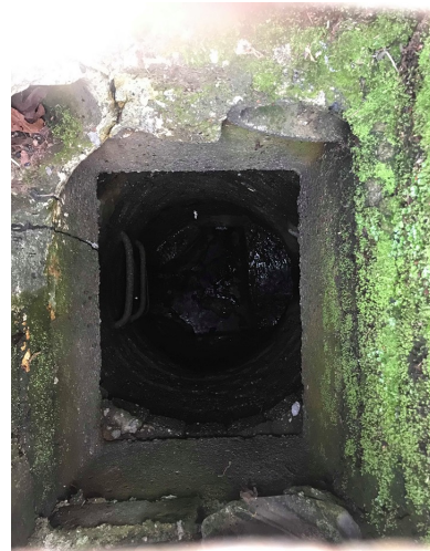
Photo 11 (looking into Type 2 CB #4): Type 2 CB (#4). 12" concrete pipe flowing east.
