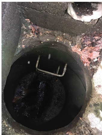
Photo 9 (looking into MH #3): Type 2 Manhole (#3). 12" concrete pipe inlet flowing north.
