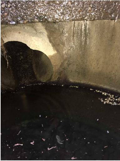
Photo 7 (looking into CB #2): Type 2 CB (#2). North outlet from 12" concrete pipe.
