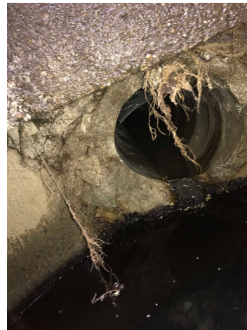
Photo 5 (looking into CB #2): Type 2 CB (#2). South inlet from 12" concrete pipe.
