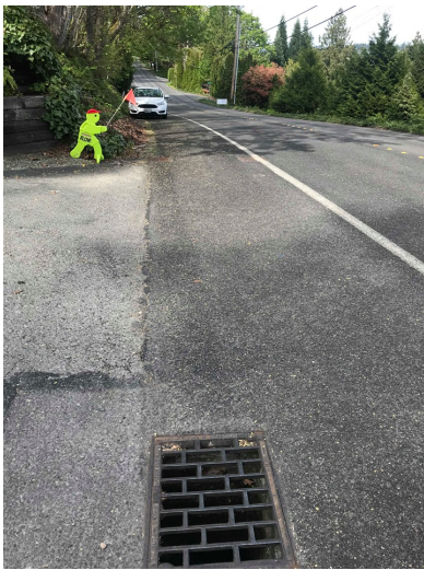
Photo 3 (looking N): Type 2 Catch basin (#2).
