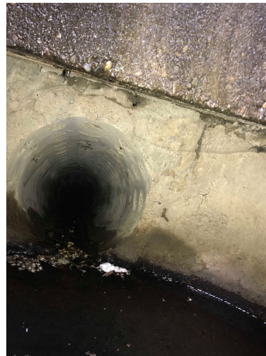
Photo 6 (looking into CB #2): Type 2 CB (#2). East inlet from 12" concrete pipe.
